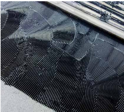
Fig. 12 Sikaflex®-298 applied with a comb spreader
