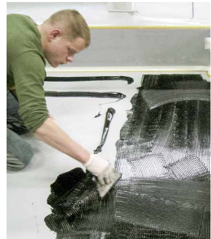
Fig. 55 Application of Sikaflex®-298
