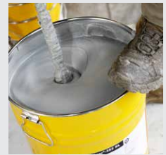
Fig. 5 Mixing SikaTransfloor®-352
