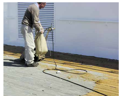
Fig. 20 Sanding the deck
