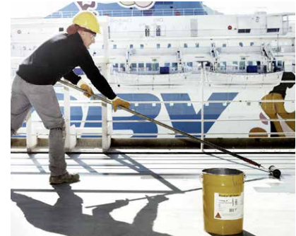
Fig. 3 Applying SikaCor® ZP Primer with a roller
