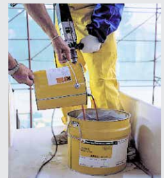
Fig. 6 Transferring the SikaTransfloor®-352 (SL/ST) to another container
