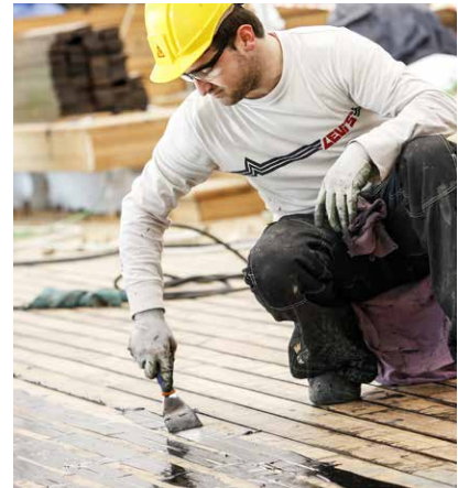
Fig. 19 Compressing Sikaflex®-290 DC PRO with a spatula
