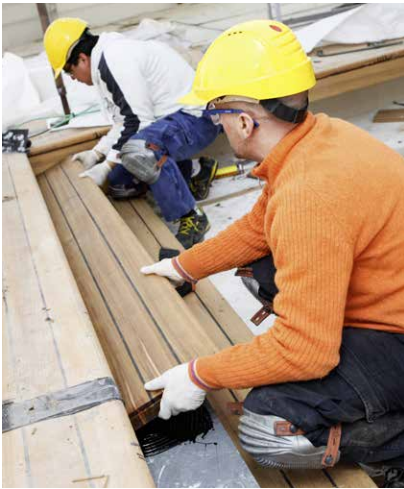
Fig. 13 Putting down the decking
