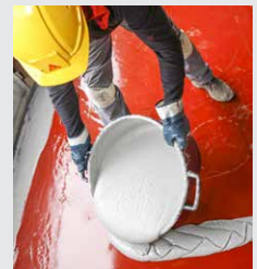
Fig. 7 Pouring the SikaTransfloor®-352 (SL/ST) to the floor
