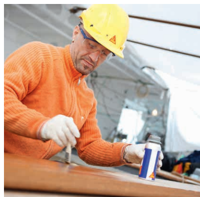
Fig. 10 Carefully applying Sika® Primer-290 DC or Sika® MultiPrimer Marine
