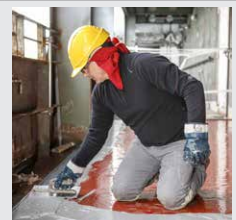
Fig. 8 Spreading the SikaTransfloor®-352 (SL/ST)
