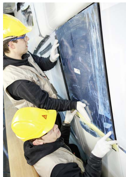
Fig. 7 The window is fitted
