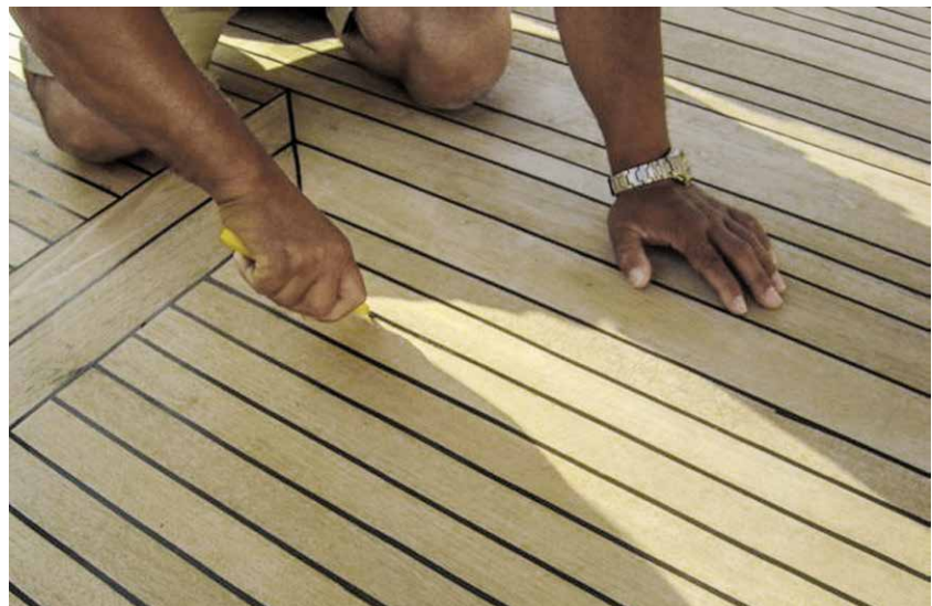
Fig. 34 Using a craft knife to cut along the part of the joint to be removed
