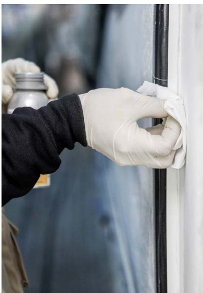
Fig. 5 Pre-treatment of the ceramic ink area with Sika® Aktivator-100
